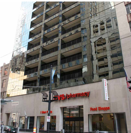
Kirby Building today.
