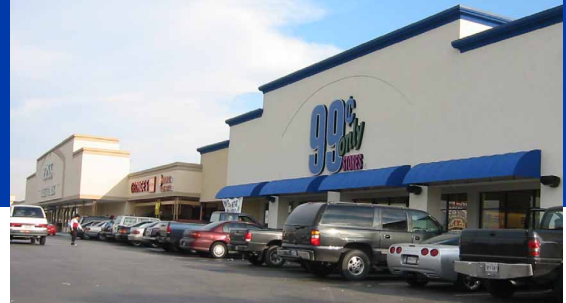
116,000 sf center (95% occ.) at Chimney Rock & Westheimer – Total imps assessed at $100.00.
